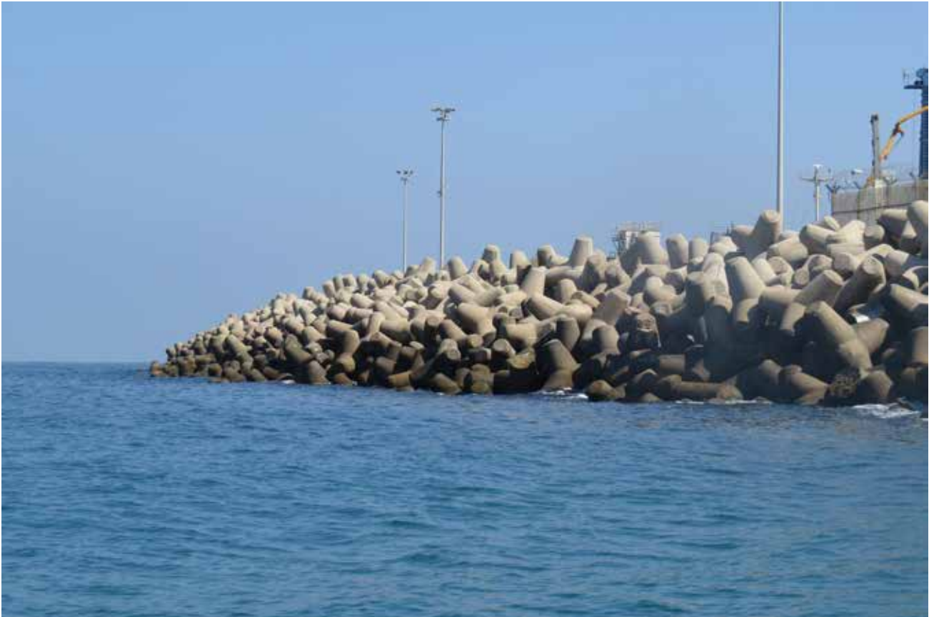
Fig 32: Ashdod port wave breaker
